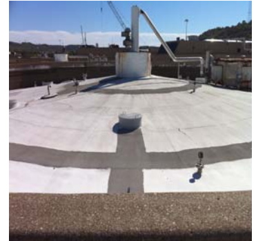
Anaerobic Digester at Mill Creek Wastewater Treatment Plant
